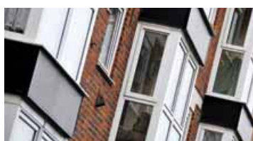
Figure 16 AIB exterior painted panel
