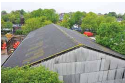
Figure 32 Asbestos cement roof and wall cladding
