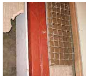
Figure 21 AIB column fire protection in CLASP building
