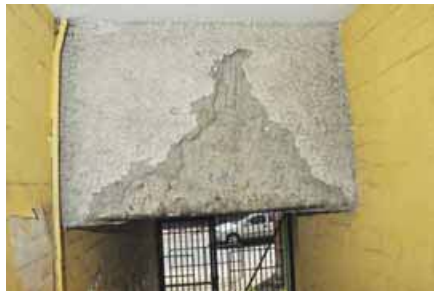
Figure 8 Sprayed coating on building passageway
