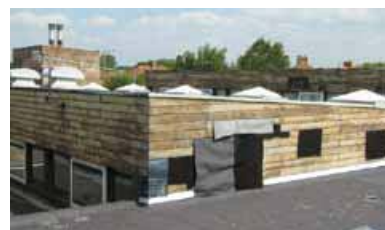
Figure 23 AIB fascia panels with wood effect finish
