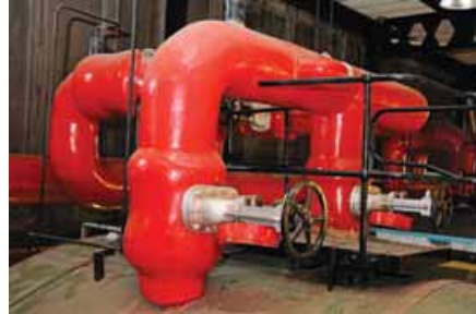
Figure 48 Asbestos-insulated supply pipes
