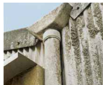
Figure 35 Asbestos cement downpipe
