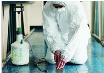
Spray water under the tiles to suppress dust as you lift them gently, avoiding breakage
