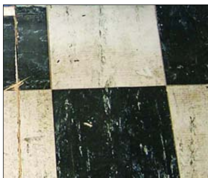
Floor tiles that contain asbestos can also have asbestos-paper backing, or be fixed with asbestos-containing mastic
