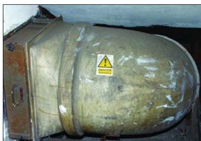
This section of AC ducting has already been labelled
