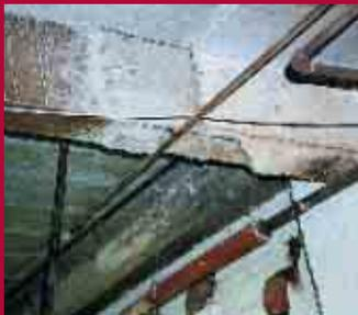
Sprayed asbestos insulation on steel framework
