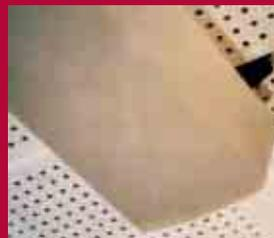
Damaged asbestos insulating board ceiling tiles
